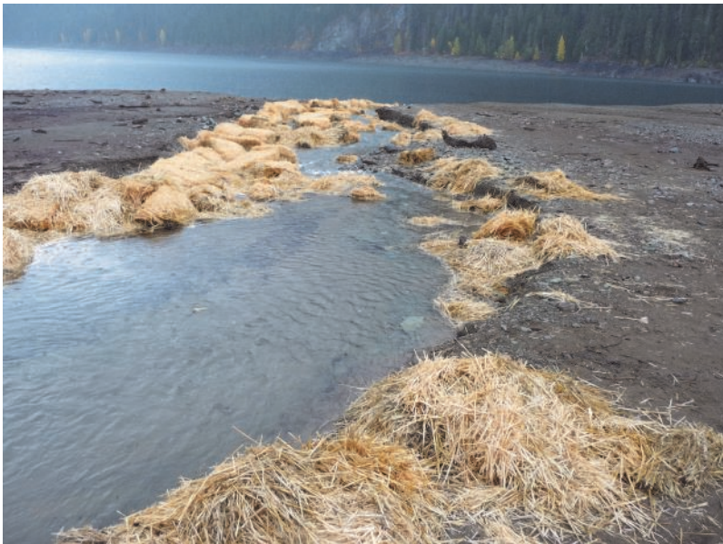
Bales of straw placed by the U.S. Bureau of Reclamation where Box Canyon Creek channel enters upper Kachess basin.
