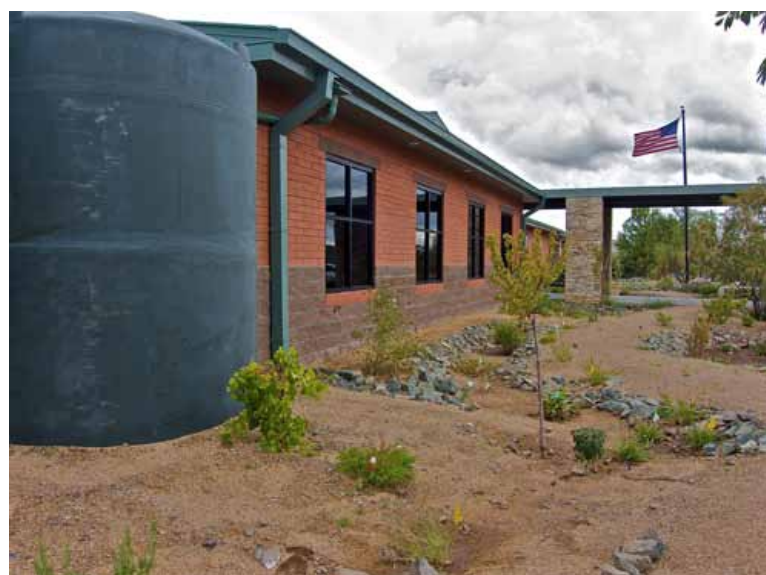
Rainwater harvesting system with drought-tolerant landscape in Prescott.
