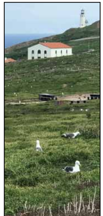
The famed lighthouse first built in 1912 got a modern upgrade in 1932 and still guides sailors through the SB Channel.
