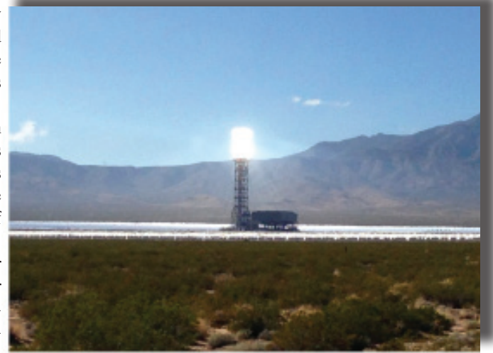
One of the Ivanpah towers operating. The intense heat from tens of thousands of mirrors creates a huge heat field deadly to birds and gives the receiver atop the tower an intense flow visible for 30-50 miles.
