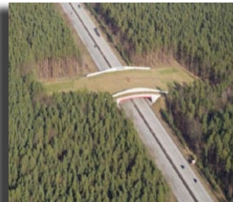
A wildlife overpass on Highway 93 in Montana (Image via Big Think) http://www.planetexperts.com/montanas-wildlife-crossings-keep-animals-off-highway-93/
