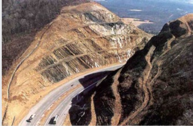
Interstate 68, 340 foot deep notch in Sliding Mountain, Maryland
