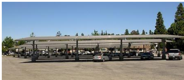
Solar awnings for parking at Taft High School in San Fernando Valley Photo by Gayle Dufour.
