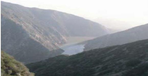
The Pacoima Reservoir that catches rain water in the mountains. (Photo NPS & The River Project)
