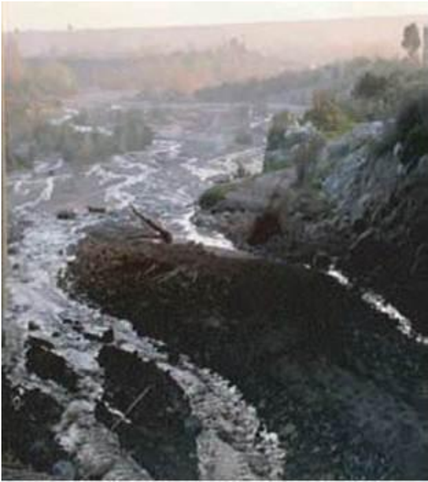
Little Tujunga Creek passes beneath the 210 Fwy; it shows the large amount of water that can come down from the mountains when it rains & snows. The intention is to capture this water to put in the underground aquifers. (Photo from The River Project)
