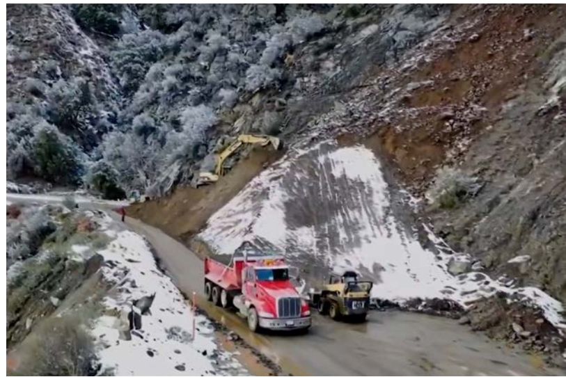
Landslide removal
