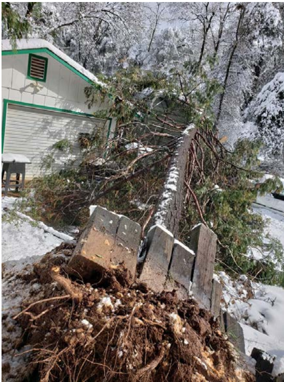
Downed tree on a house
