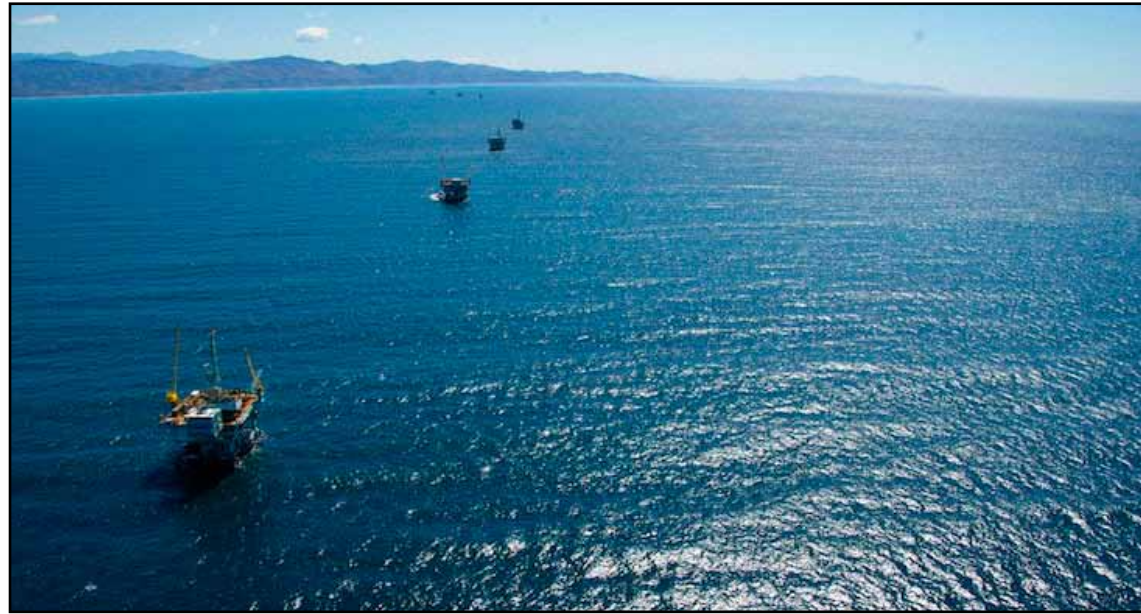
Santa Barbara Channel oil rigs are already past their expected life span and moves to 'decommission' them are underway. No word yet whether their bottoms will become artificial reefs. (Photo courtesy of BOEM)
