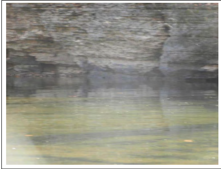
Figure 5.0.1 – Bedding planes and vertical fractures of the bedrock adjacent to the Greenbrier River near the proposed MVP crossing. Bedrock is also present in the river bed.
