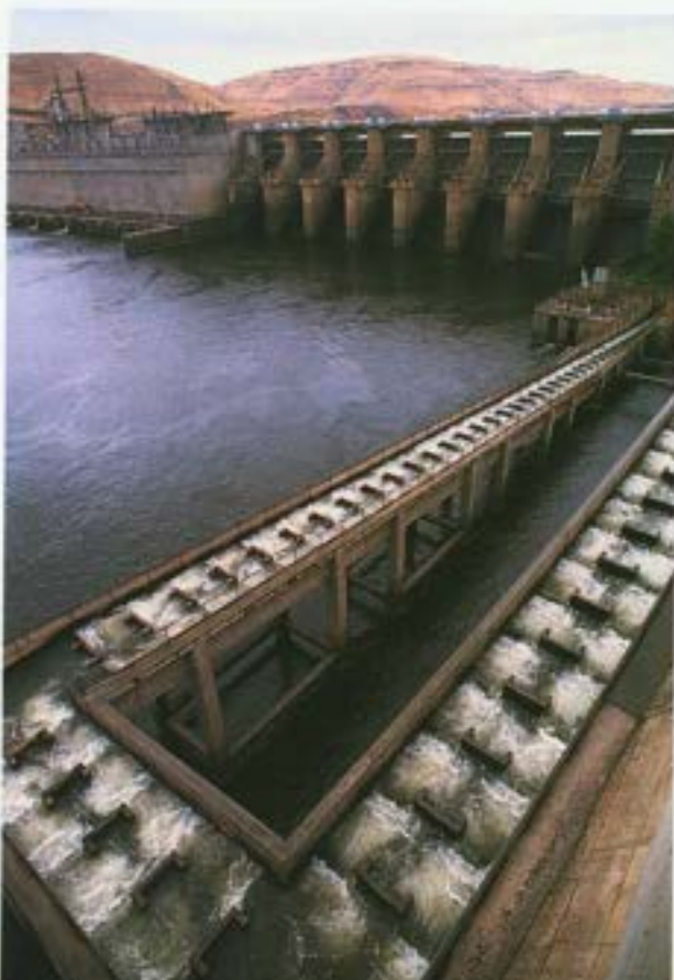
Bonneville Dam (facing page) is the first hurdle for returning salmon. Below, a fish ladder on Lower Monumental Dam.
