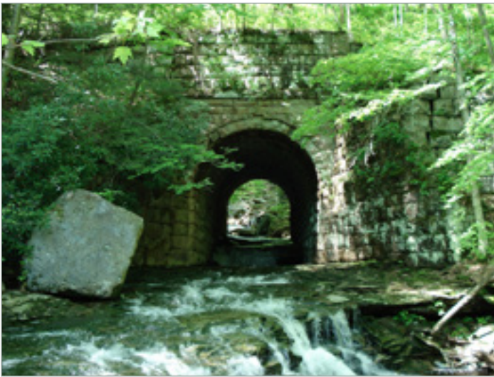
Blackwater Canyon Trail Culvert at Big Run Tributary PHOTO: PUBLIC DOMAIN.
