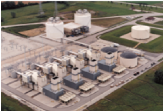
WE Energies' Paris Generating Station in Union Grove: A natural gas based combustion turbine plant. www.we-energies.com/company/pdf/Paris.pdf
