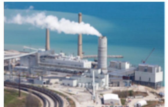
The Oak Creek plant occupies 1,000 acres of lakeshore and uses an average of 6,000-6,200 tons of coal daily. www.we-energies.com/company/pdf/oak-creek-power-plant.pdf
