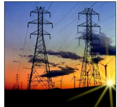
Transmission lines. Photo Credit: National Renewable Energy Laboratory
