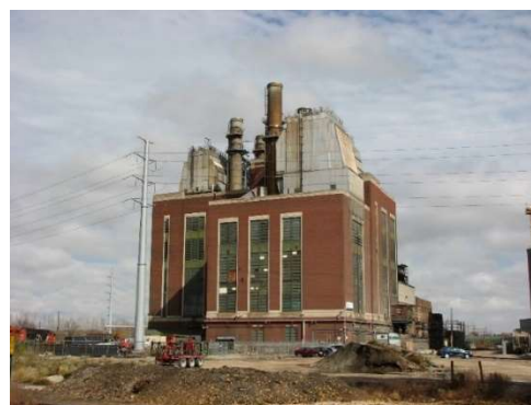
Sixth Street Generating Station. Photo by Elwood Garlock.
