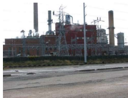
Prairie Creek Generating Station. Photo by Elwood Garlock.
