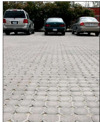
Permeable pavement. Photo by Jason Johnson, USDA NRCS
