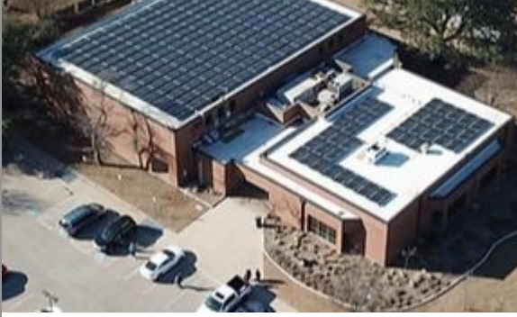
Solar panels on Fretz Park Recreation Center
