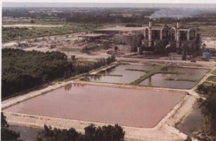
This Dade County, Fla., incinerator removes many recyclables before burning waste, but it does not employ scrubbers to reduce smokestack emissions.
