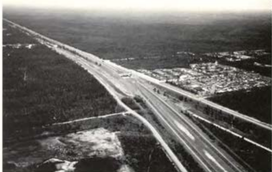
Today, more than two decades after ground was broken for southwest Florida's Golden Gate Estates subdivision, only a fraction of the original site has been fully developed. The canals that were dug to drain this swampy land caused local water tables to drop dramatically.
