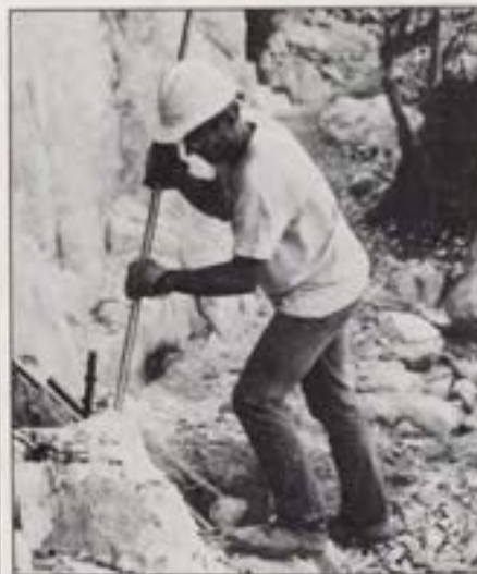
Goodale Pass Trail work, Sierra (Sandy Gimbal)
