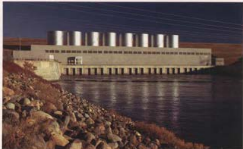
Millions of acre-feet of Missouri River water would be diverted by projects on the drawing board or already completed (such as the Ft. Randall Dam, above, in South Dakota).
