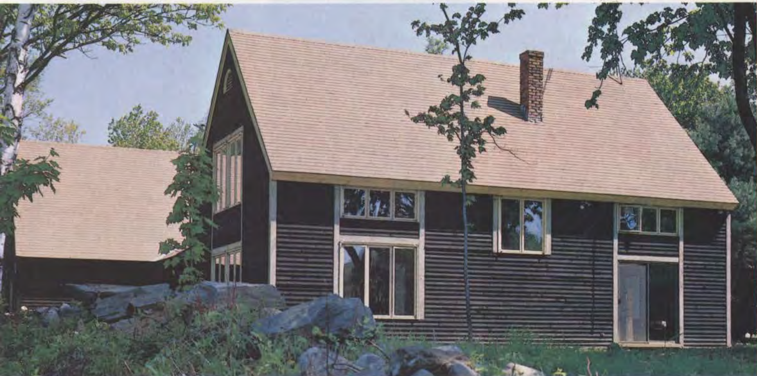
This prefabricated passive solar home, resembling a New England barn, is ideal for its rustic Vermont setting. The house combines direct- and indirect-gain systems and a wood-burning stove to defeat New England winters. Maple and birch trees shade the house in the summer months but don't block the sun's rays in winter.
