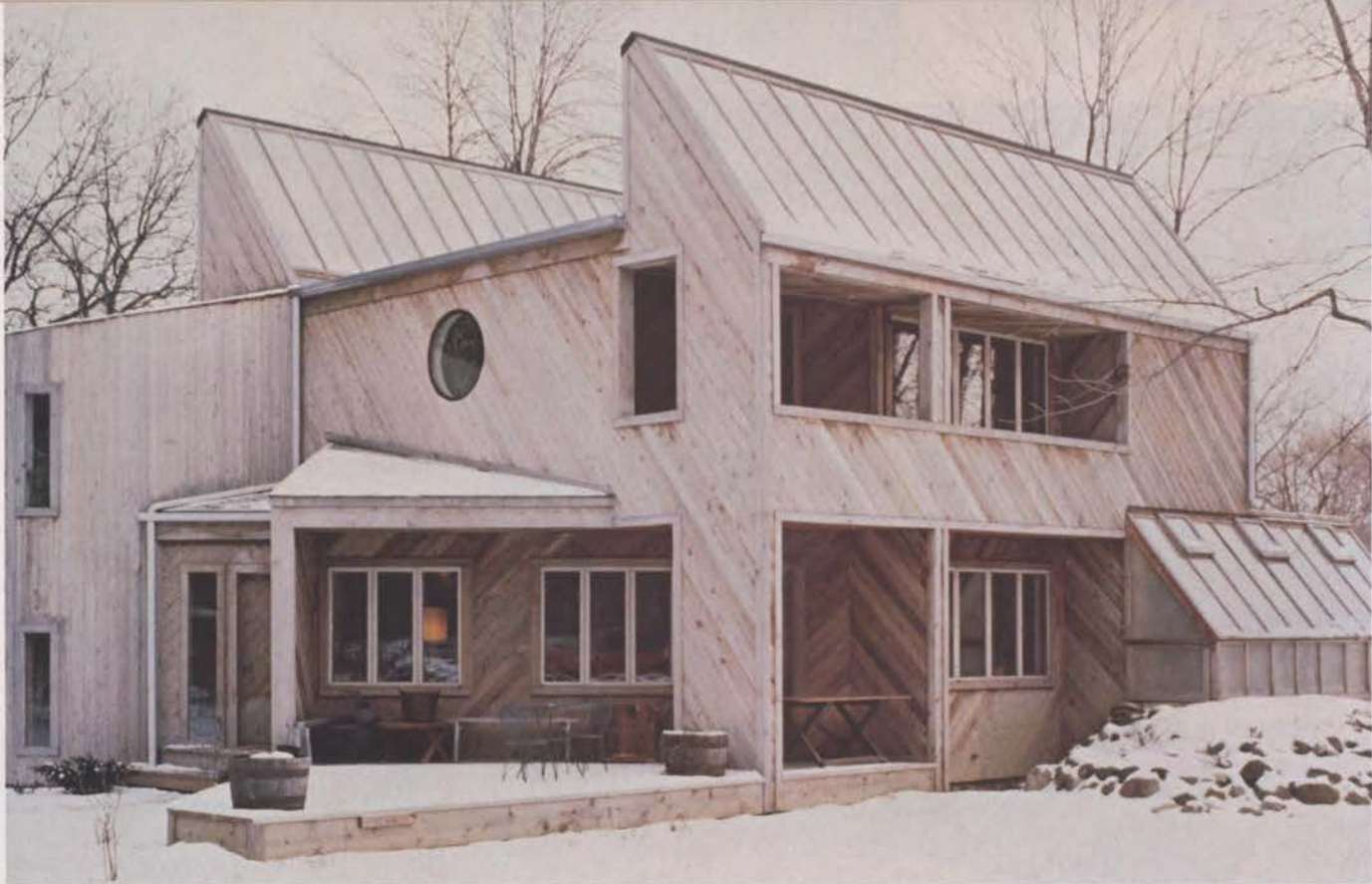
A snow-covered landscape, overcast sky and temperatures below zero don't negate the efficiency of this solar heating system. Sun is drawn into the house through south-facing windows, a greenhouse and rooftop collectors.
