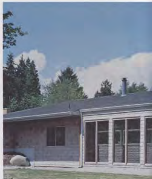
Thermal storage wall of bricks, faced by glass, forms the backbone of this house's passive solar system. Vents in the gravel floor can be adjusted to regulate the flow of air into the heating chamber.
