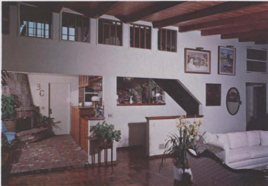
Windowlike openings just below the ceiling form an integral part of the passive heating and cooling system, allowing a free flow of air. Circulation in the main part of the house is also aided by the open floor plan, which provides easy access to all the living areas.
