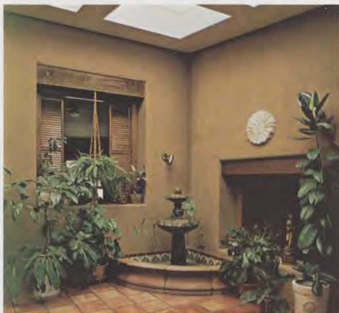
Central atrium helps keep the Duncan house warm in winter by storing solar heat in the adobe walls and terra-cotta floors. The skylights, which open for ventilation during the summer, can be screened to block sunlight when it's unwanted. Shuttered doors permit air circulation between rooms.
