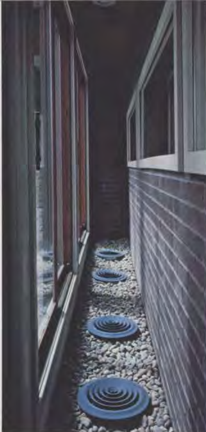
Thermal storage wall of bricks, faced by glass, forms the backbone of this house's passive solar system. Vents in the gravel floor can be adjusted to regulate the flow of air into the heating chamber.
