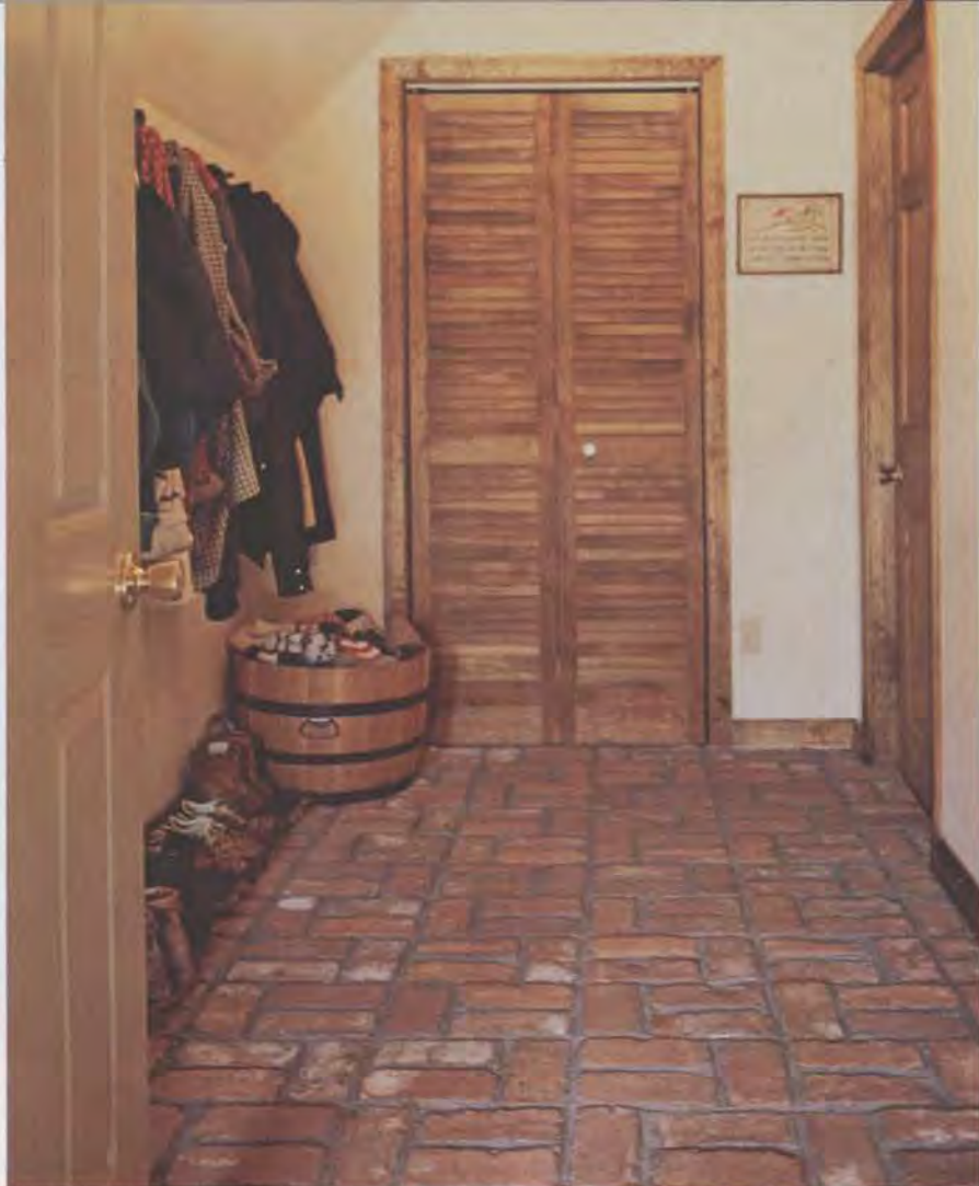
Brick-floor foyer acts as a buffer to moderate outside temperatures. Extreme heat loss or gain is lessened because interior living areas are not directly affected by the opening and closing of the front door.
