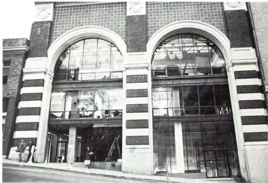
and nearing completion.
