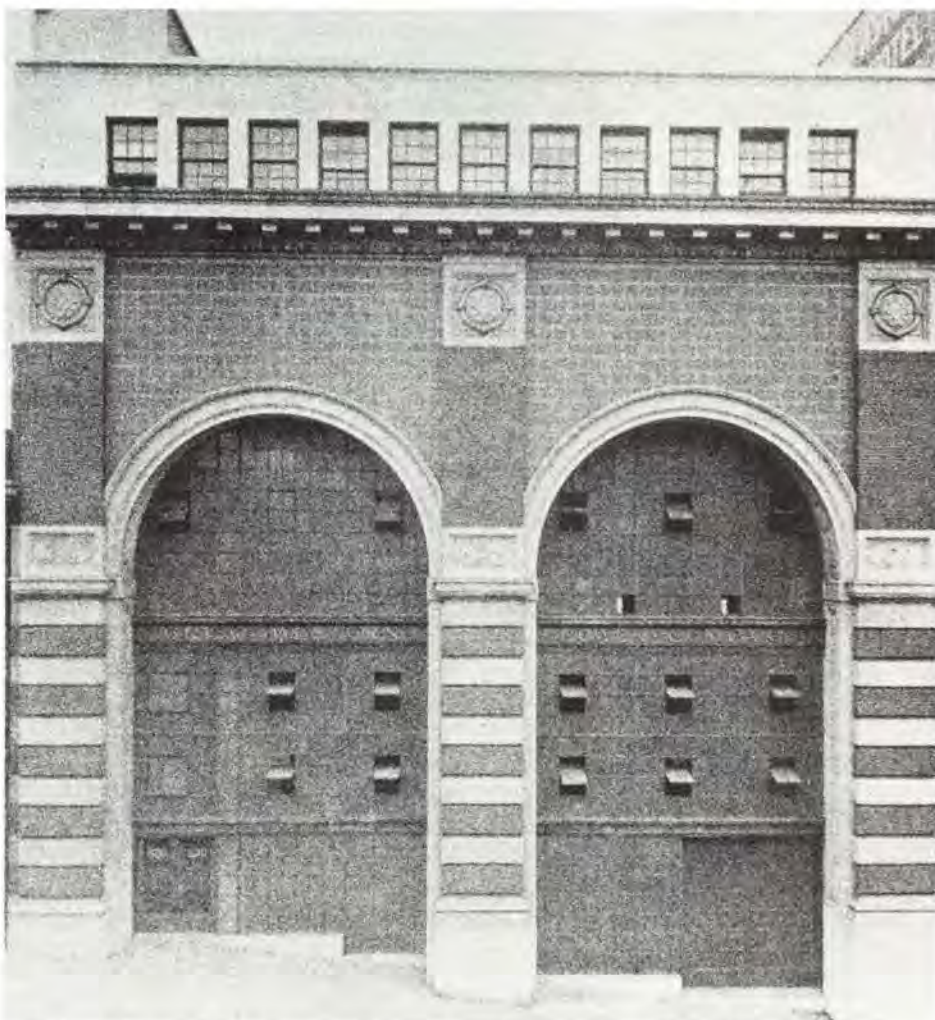
The Great Western Power Company's downtown plant as it appeared in 1916 . . .
