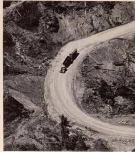
East slope. . . . A logging truck winds through the devastated, unstable land.
