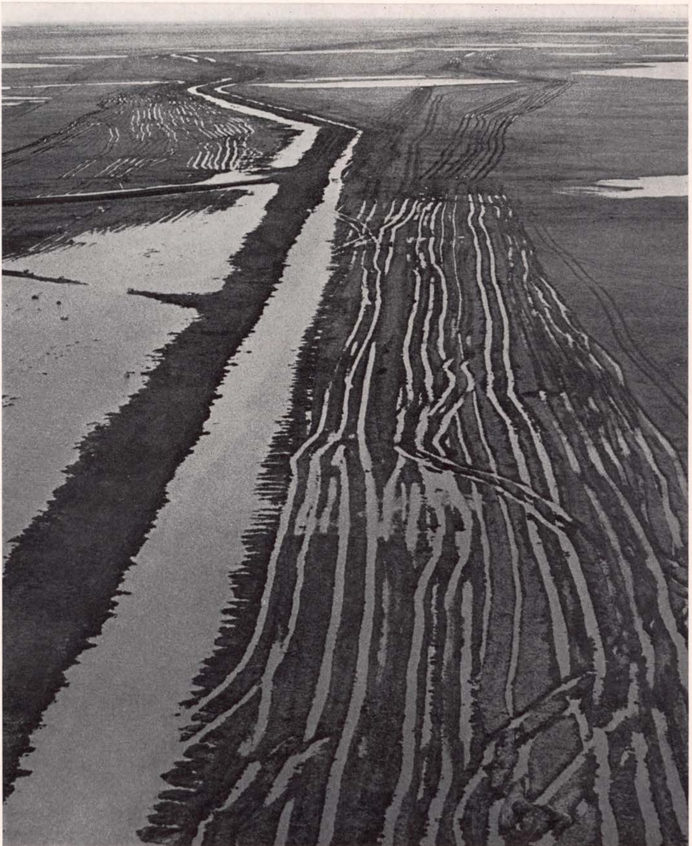
On the trail of a caterpillar. Road building in the Arctic: scrape the tundra into a mound, expose the perma-frost, and the result is instant rivers.
