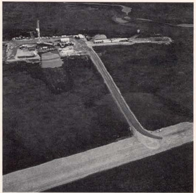
Gravel for construction pads and runways like this . . .
