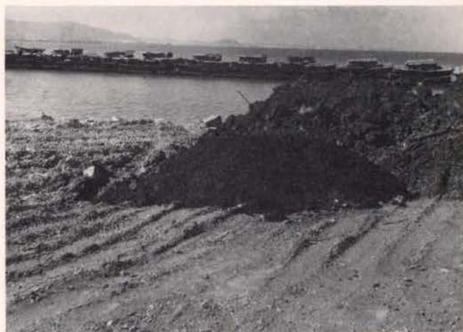
Burlingame's Bay fill project is typical of many around the shoreline; dikes mark out the area slated for fill, and dirt piles accumulate in preparation for bulldozing. Photo by Susan Landor.
