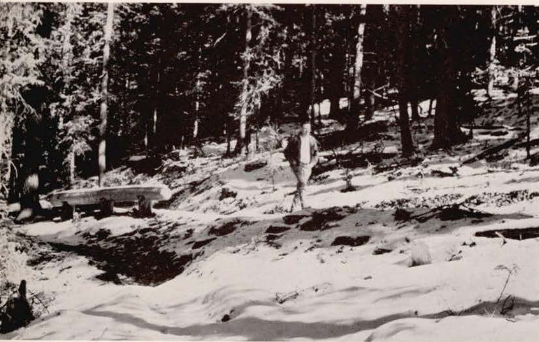
Hiker strolls 120 feet to gain four feet in elevation on over-engineered Trampas Trail, Pecos Wilderness Area, New Mexico. Note massive barrier intended to discourage shortcutting. Photo by Stanley E. Logan.
