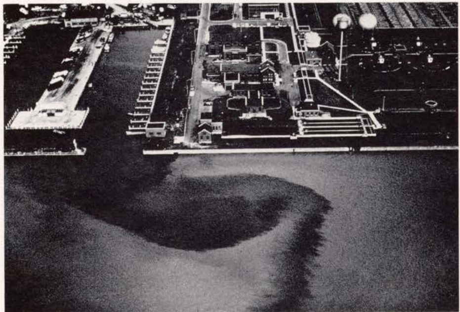
Sewage treatment plant at Toledo discharges effluent into Maumee River.
