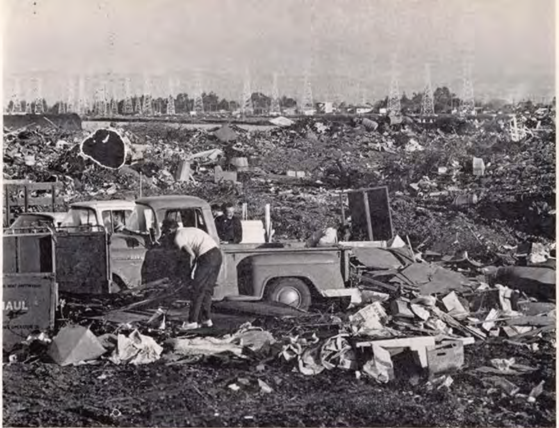
San Mateo dump. Photograph by Rondal Partridge.
