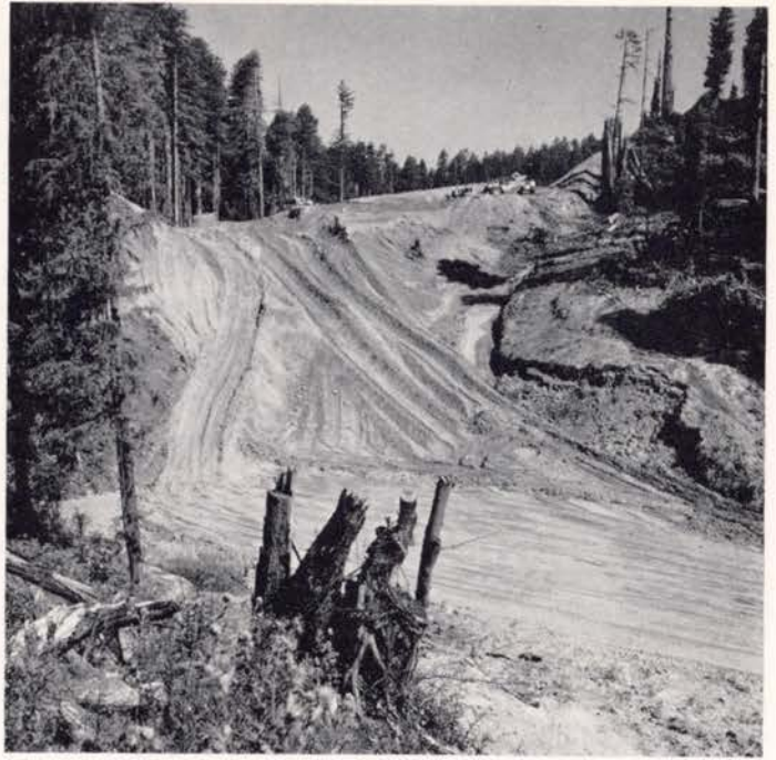
Freeway Construction North of Prairie Creek
