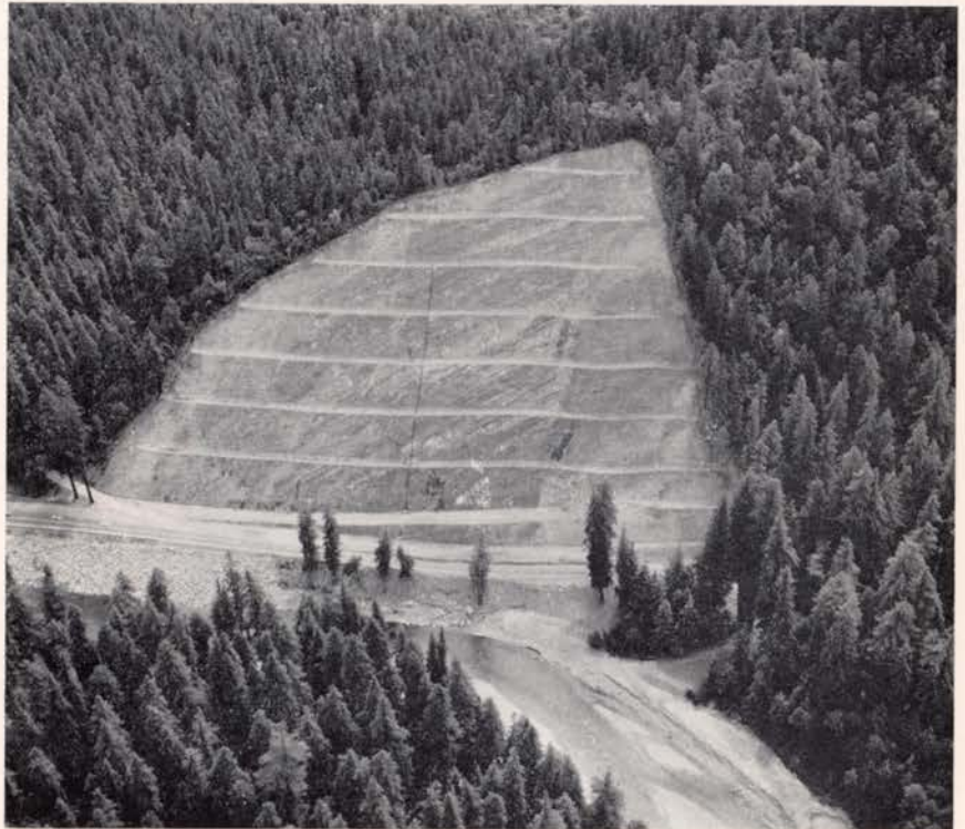
The Division of Highways caption for this photograph reads as follows: "View of the famous high cut near the Federation of Women's Clubs Grove in the Humboldt Redwoods State Park. The uppermost part of the cut is 480 feet above the roadbed. South Fork Eel River is in the foreground."
