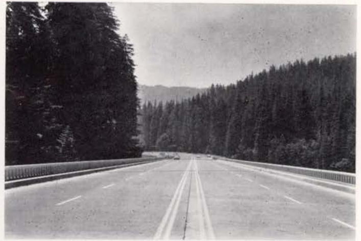
Freeway bridge over the South Fork of the Eel River at Founder's Grove in Humboldt Redwood State Park. Photograph by Philip Hyde.
