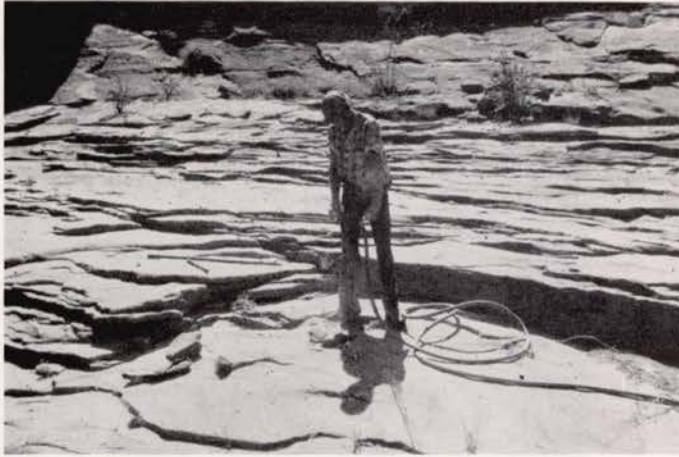
In Aztec Canyon near its junction with Bridge Canyon, a few miles below Rainbow Bridge, a workman in May was making anchors for the new quarter million dollar floating landing described on pages 2 and 14 of the June Sierra Club Bulletin. This is part of the $16 million recreational development of the new Glen Canyon Recreation Area. Photo by David R. Toepfen
