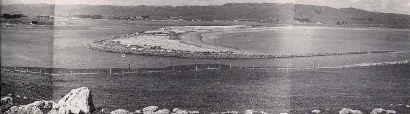
This panoramic photograph by Josephine Alexander was taken in series and stripped together to show the Doran Park sandpit at right and Bodega Head, left, with the P.G.&E. Atomic Reactor Site construction activity in the center (meteorological tower on far left to record wind directions). Scientists of the U.S. Geological Survey are now conducting an intensive inquiry into the earth formations and any indications of
