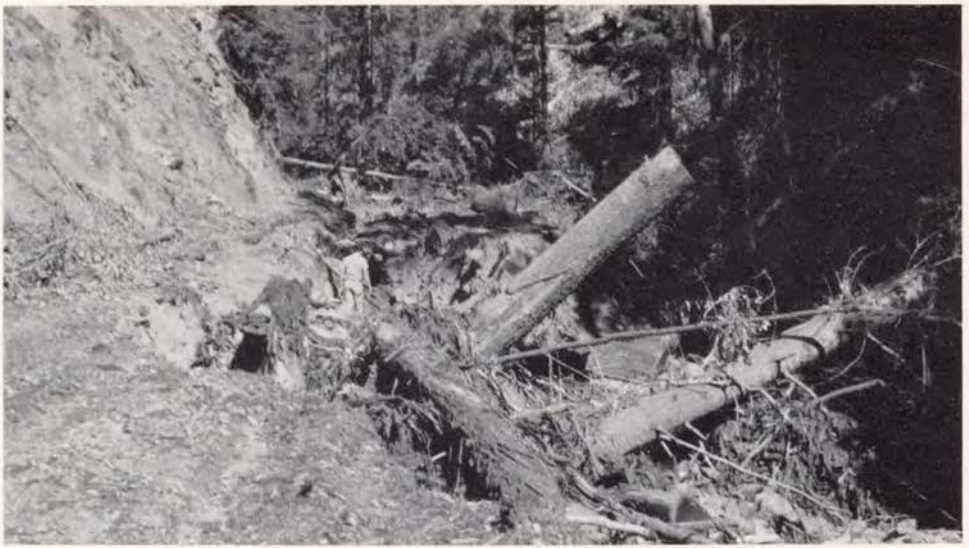
This road, built along the banks of a tributary of Pepperwood Creek in Sonoma County during a logging effort some years earlier, was eroding badly when this photograph was taken in 1962 by Charles Seeley.
