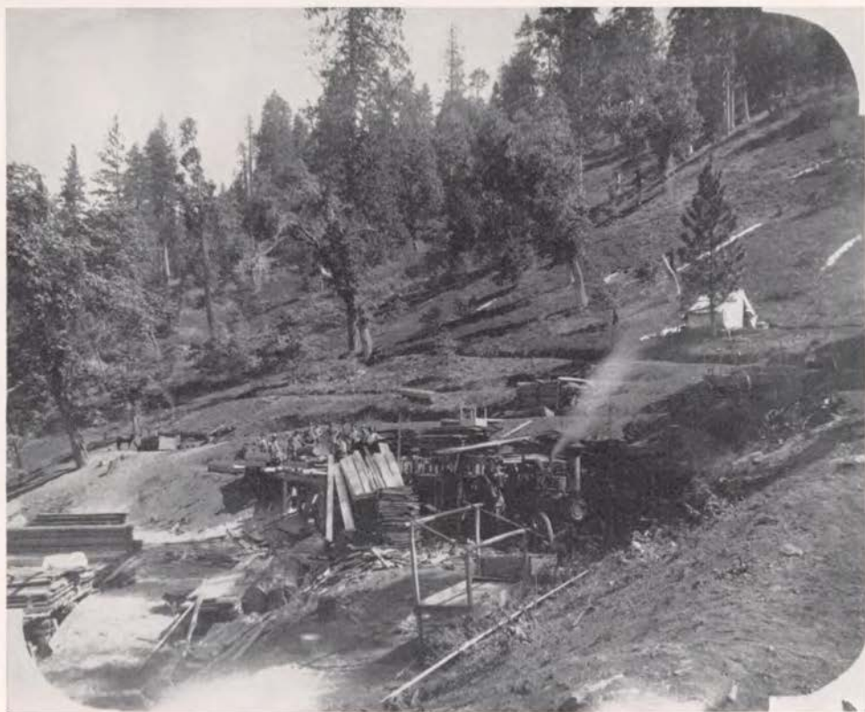
Kaweah Colony's "Ajax" in the pines, the self-propelling steam engine used to power the colonists' lumber mill. Courtesy National Archives
