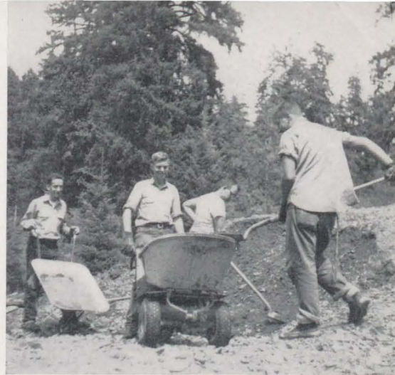
TRAIL CONSTRUCTION, Olympic National Park by Charles Maiden
