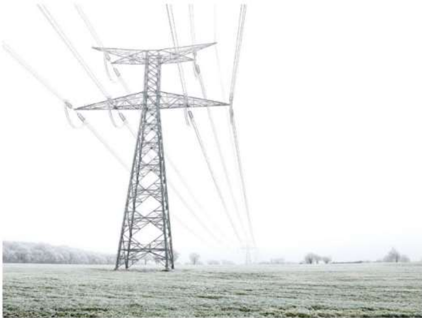
Ice covers electrical sources
