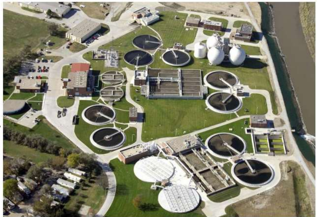
Lincoln, NE's Theresa Street Wastewater Treatment Plant
