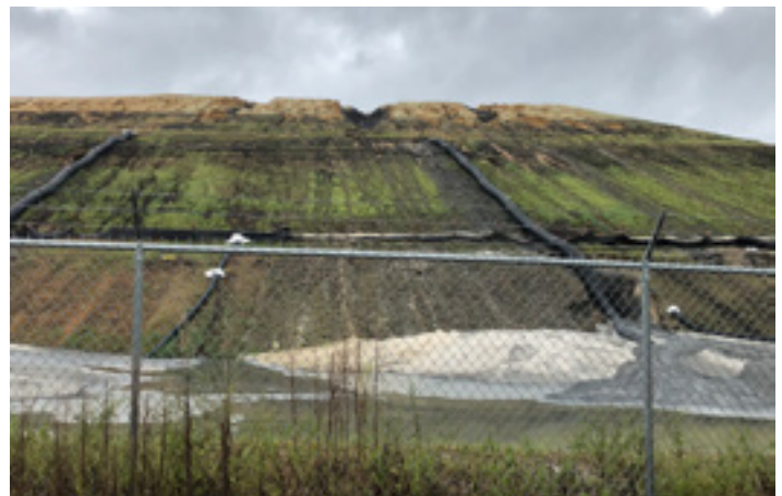
TOXIC COAL ASH IS PILED UP ABOVE THE CAPE FEAR RIVER IN UNLINED IMPOUNDMENTS AT DUKE'S L.V. SUTTON PLANT OUTSIDE WILMINGTON, NC, AND MOST OTHER COAL AS DUMPSITES. PHOTO: CAPE FEAR RIVERKEEPER
