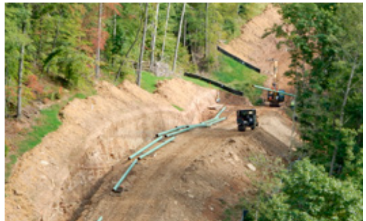
INSTALLING PIPELINE IN WEST VIRGINIA. (FEBRUARY 2016.) PROVIDED BY FRACTRACKER ALLIANCE, FRACTRACKER.ORG/PHOTOS .
