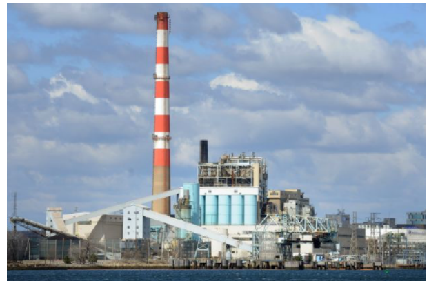
Millstone Nuclear Plant
