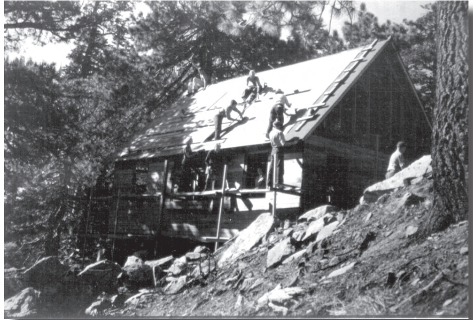
Rebuilding Baldy Hut, late 1936. Angeles Chapter Archives
