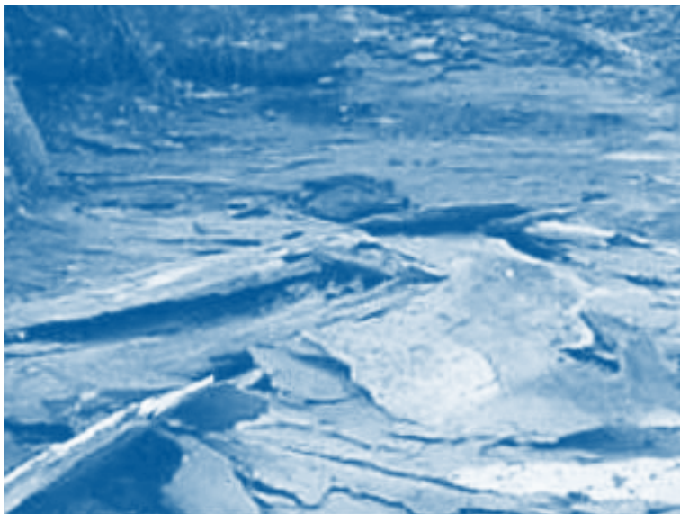
Subsidence from Longwall Mining has destructive effects across Southwestern Pennsylvania.
