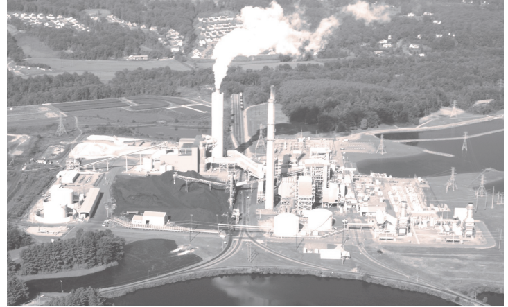
Progress Energy plant in Arden. Photo by Hartwell Carson.
