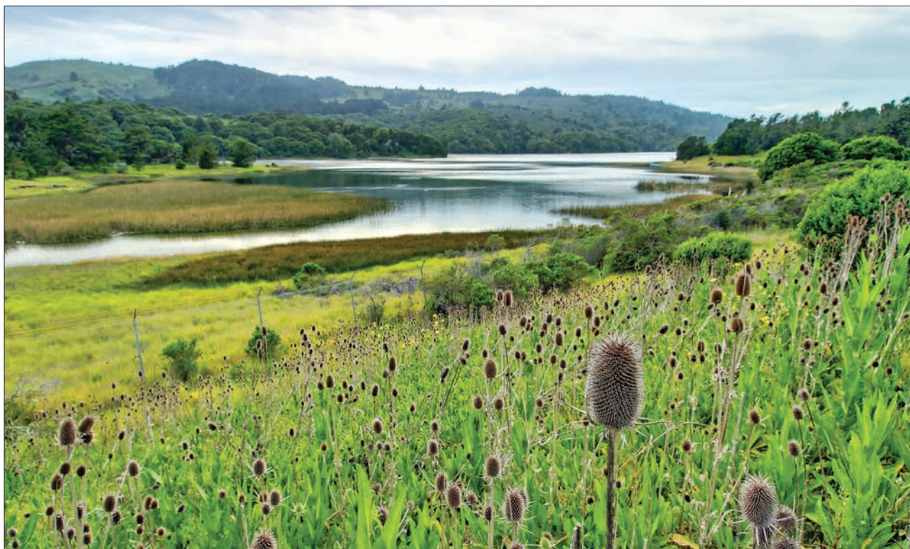
The Crystal Springs Reservoir is part of the Peninsula Watershed, a vital water source for San Francisco and suburban water districts. Photo by Chris Sagedy, http://chris.sagedy.com .
