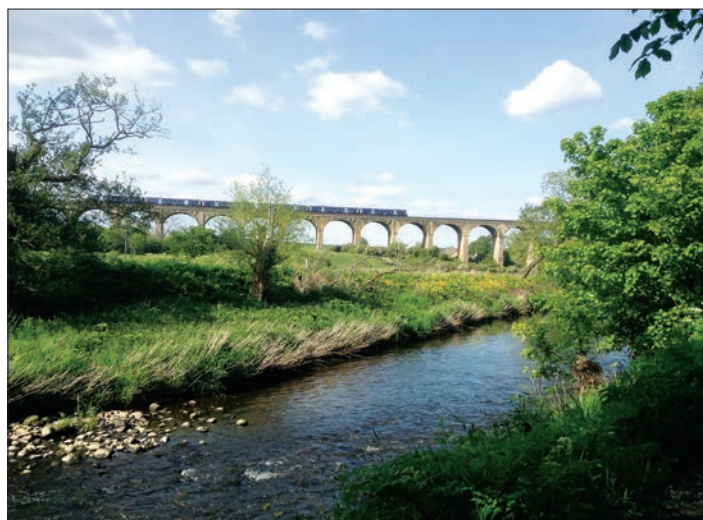
Avon Viaduct, a railway bridge in Linlithgow, Scotland. Photo by Joy Durighello.
